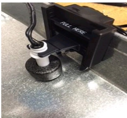
PUSH IT DOWN (SWITCH BRACKET)
