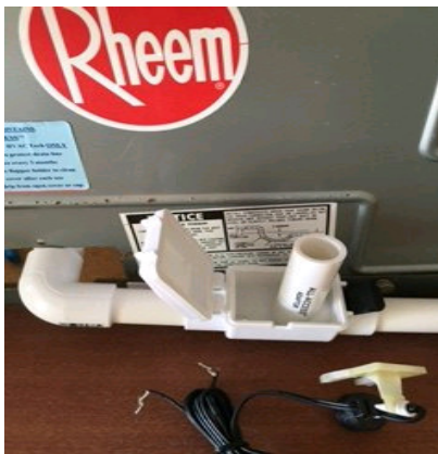
TO CLEAR DRAIN LINE INSERT THE ADAPTOR
