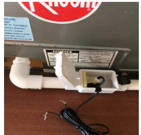
OPEN COVER TO TEST SWITCH
